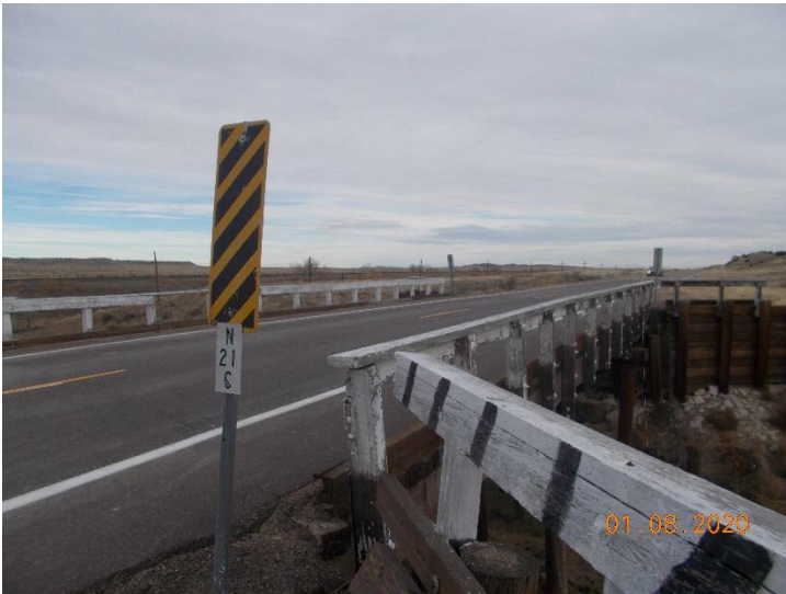
View of bridge N-21-C looking northeast.
